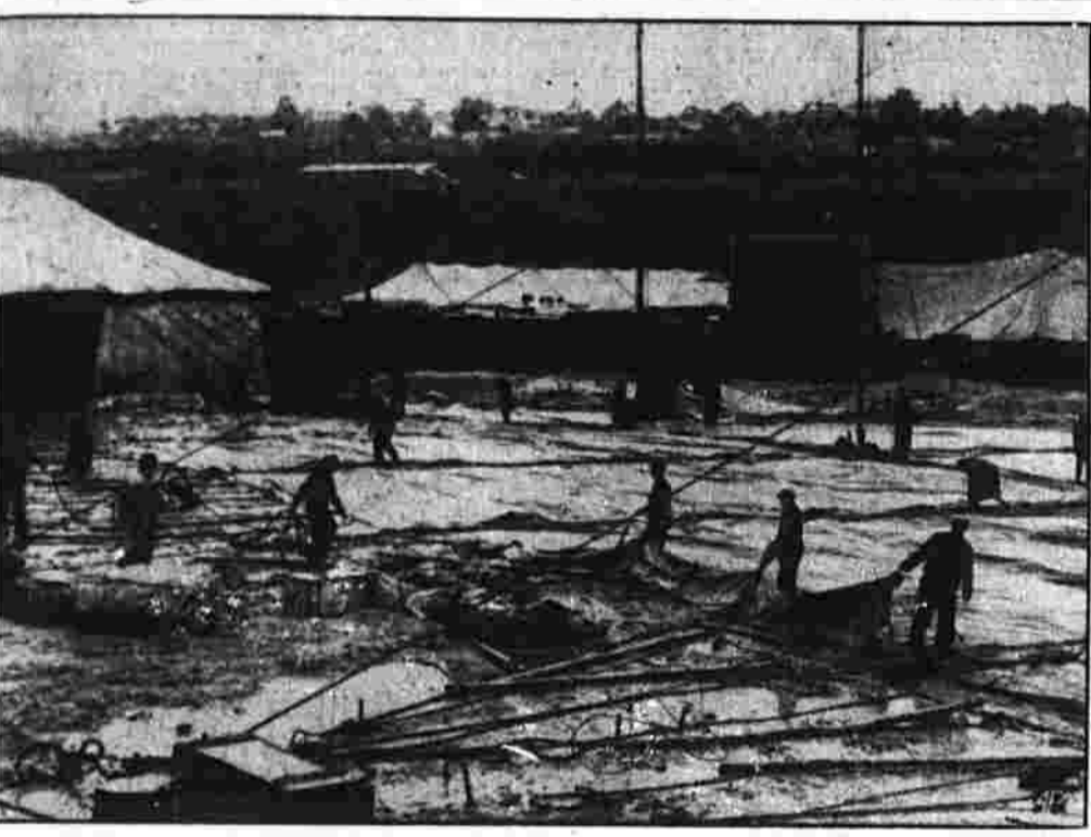
Stalled at Scranton, Pa., by rain and a strike of workmen who refused to take a wage cut, Ringling Brothers-Baron & Bailey's "Greatest Show on Earth" folded its "big Top" for the summer at an unprecedentedly early date. Here workmen are folding the canvas to ship it along with other equipment to the circus winter quarters at Sarasota, Fla.
